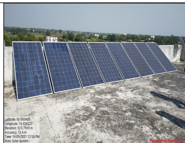
Solar Panels on Terrace (Capacity: 2 KW used for street light)
